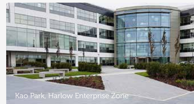
Data Campus, Harlow Enterprise Zone
